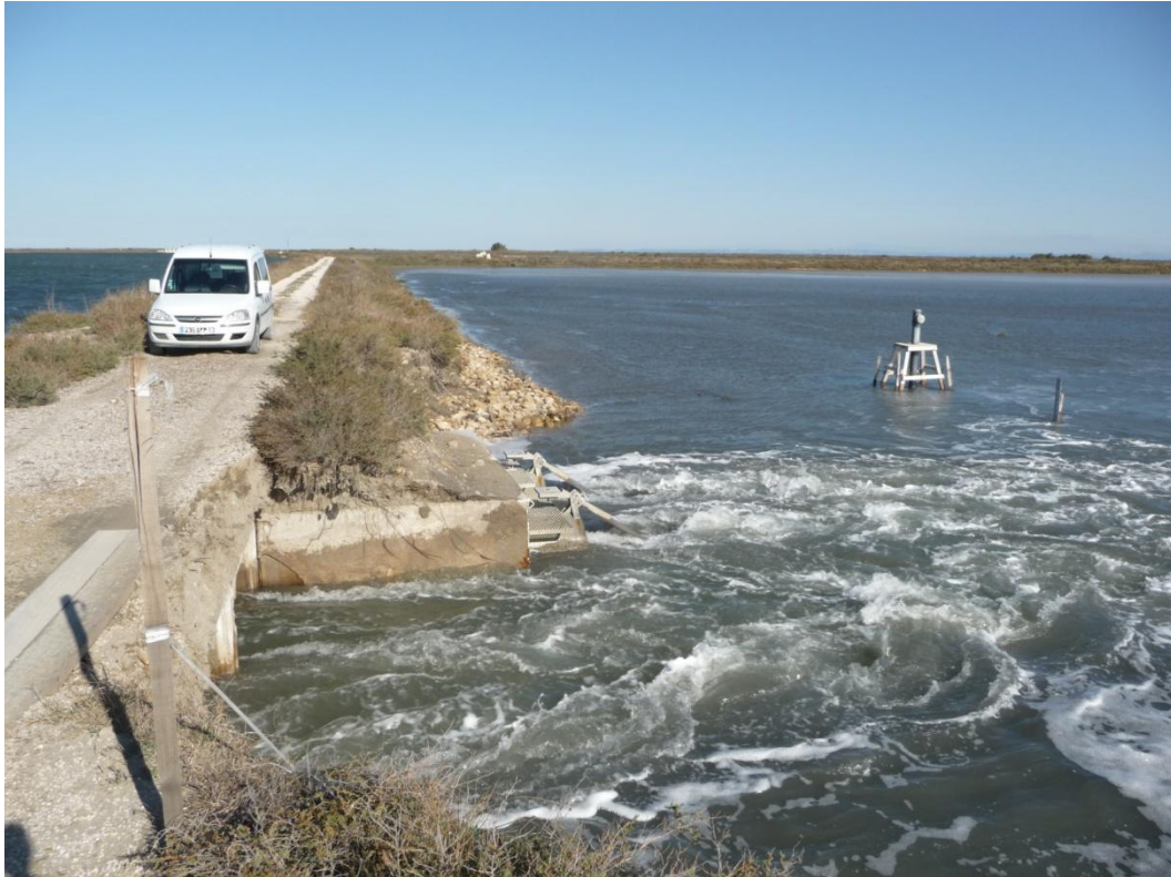
Photo 13 : Connexion Tampan/Galabert © Y. Chérain/SNPN-RNNC
