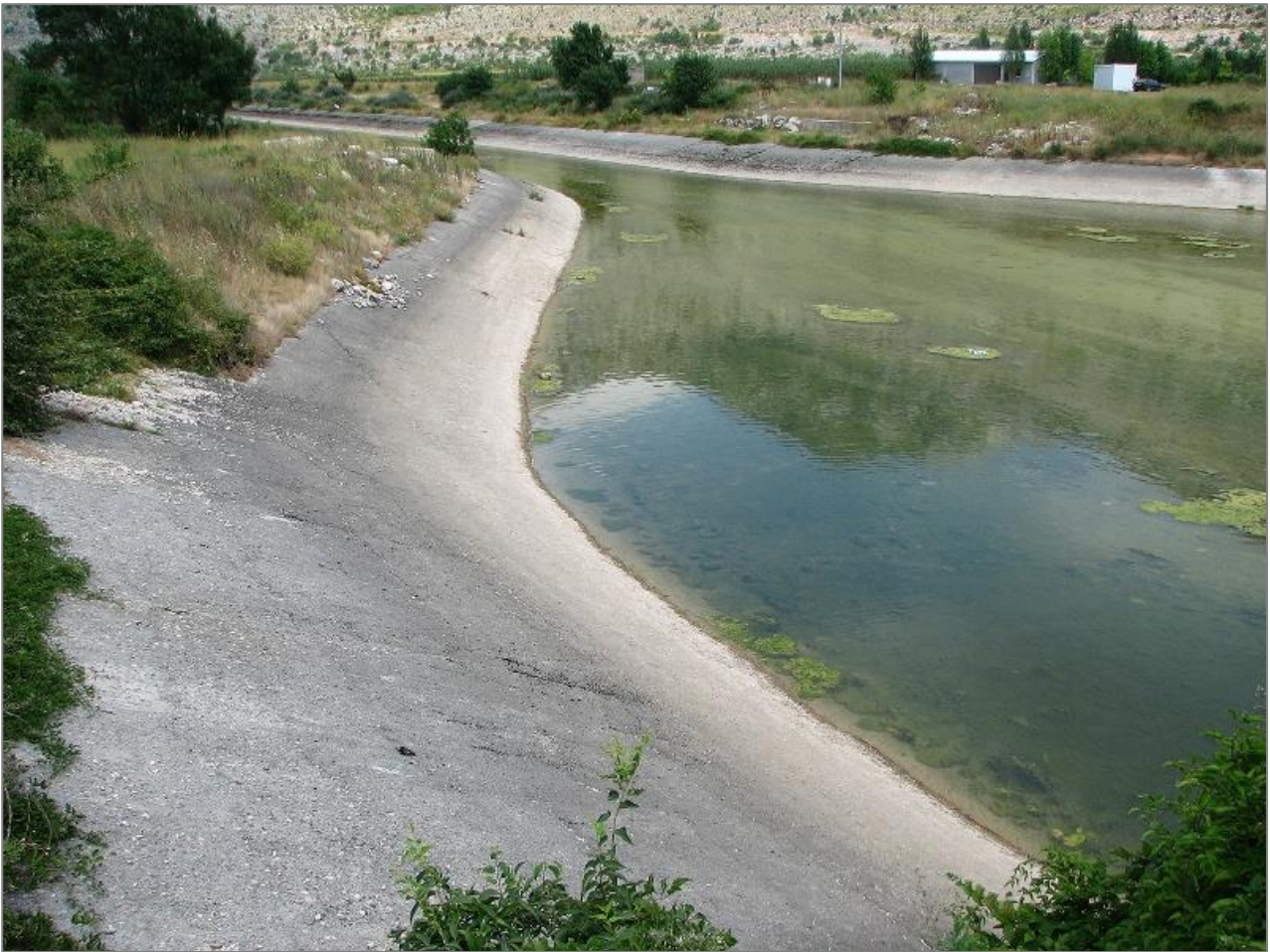
Figure 5. Trebišnjica River transformed into canal in Popovo karst polje
